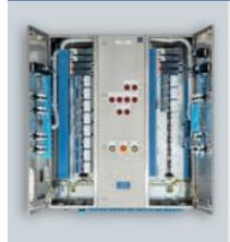
For repairs, maintenance or expansions, Ex i-protected system solutions are particularly easy to handle. Thanks to this type of protection, these tasks can be carried out during operation in hazardous areas, even when live (hot work), without having to switch off the entire system or parts of the system (hot swap).
